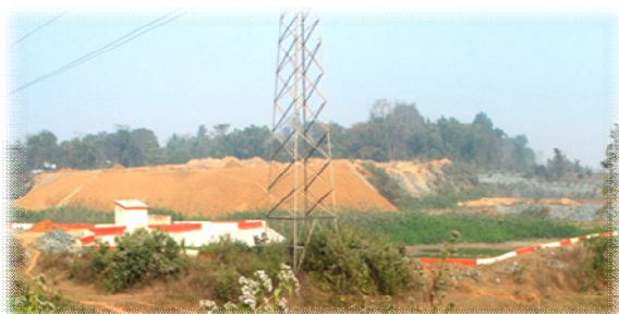
Soil covering & Garland drain around the dump
